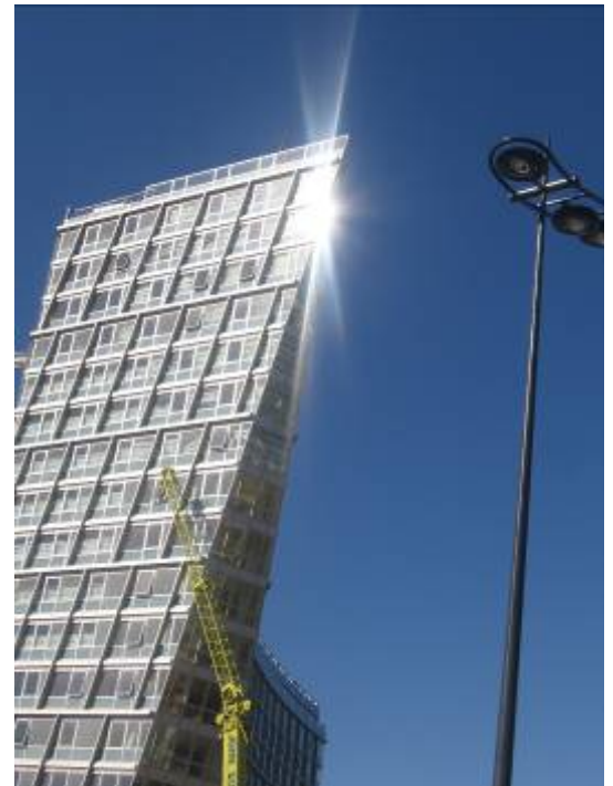
"One Park West", The Strand, Liverpool One – under construction in summer 2008
